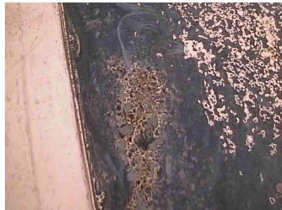
The copper sheet corrosion
