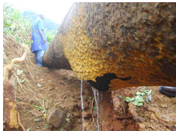
Damage of rubber coating on buried pipe
