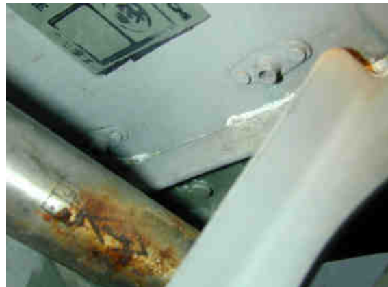
Galvanic Corrosion on the MB-339 Attach Fitting
